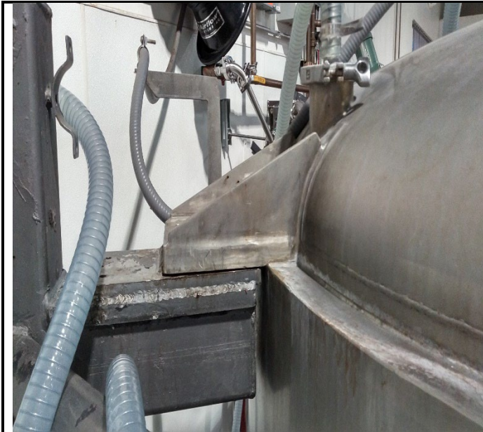
Tank welded to carbon steel frame
